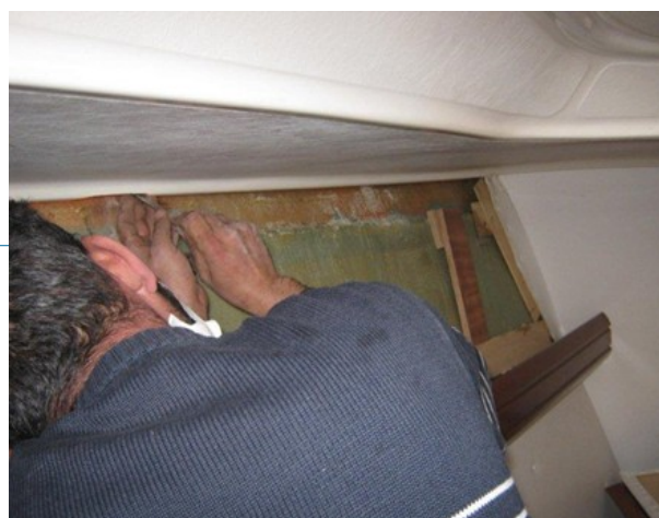
Fig 1(b) – Removing the interior lining
